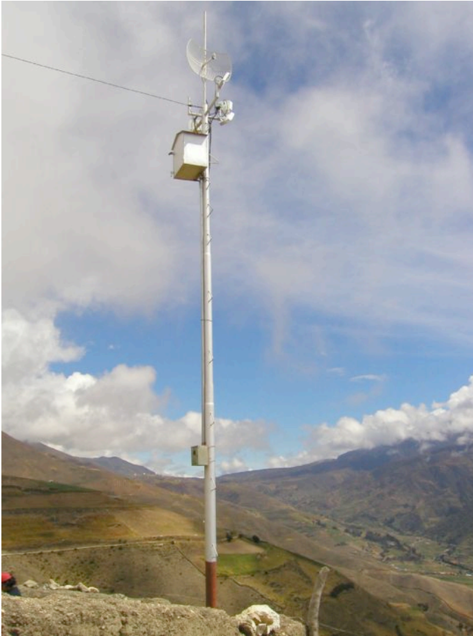
Figure 7.3: A simple self-supporting tower.
